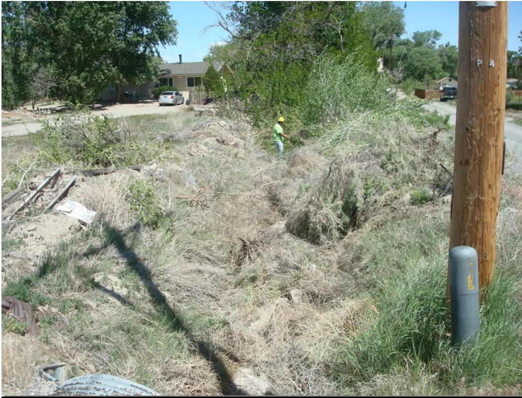
Before Construction at Irrigation Return Flow Site
