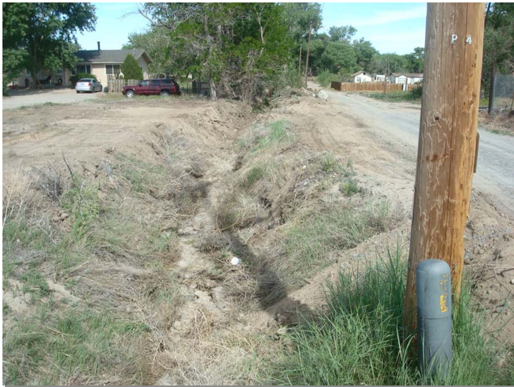
After Construction at Irrigation Return Flow Site
