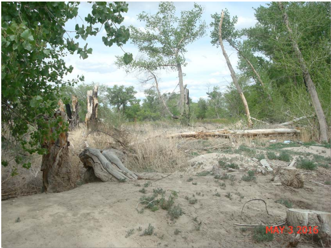
Before Construction at Irrigation Return Flow Site
