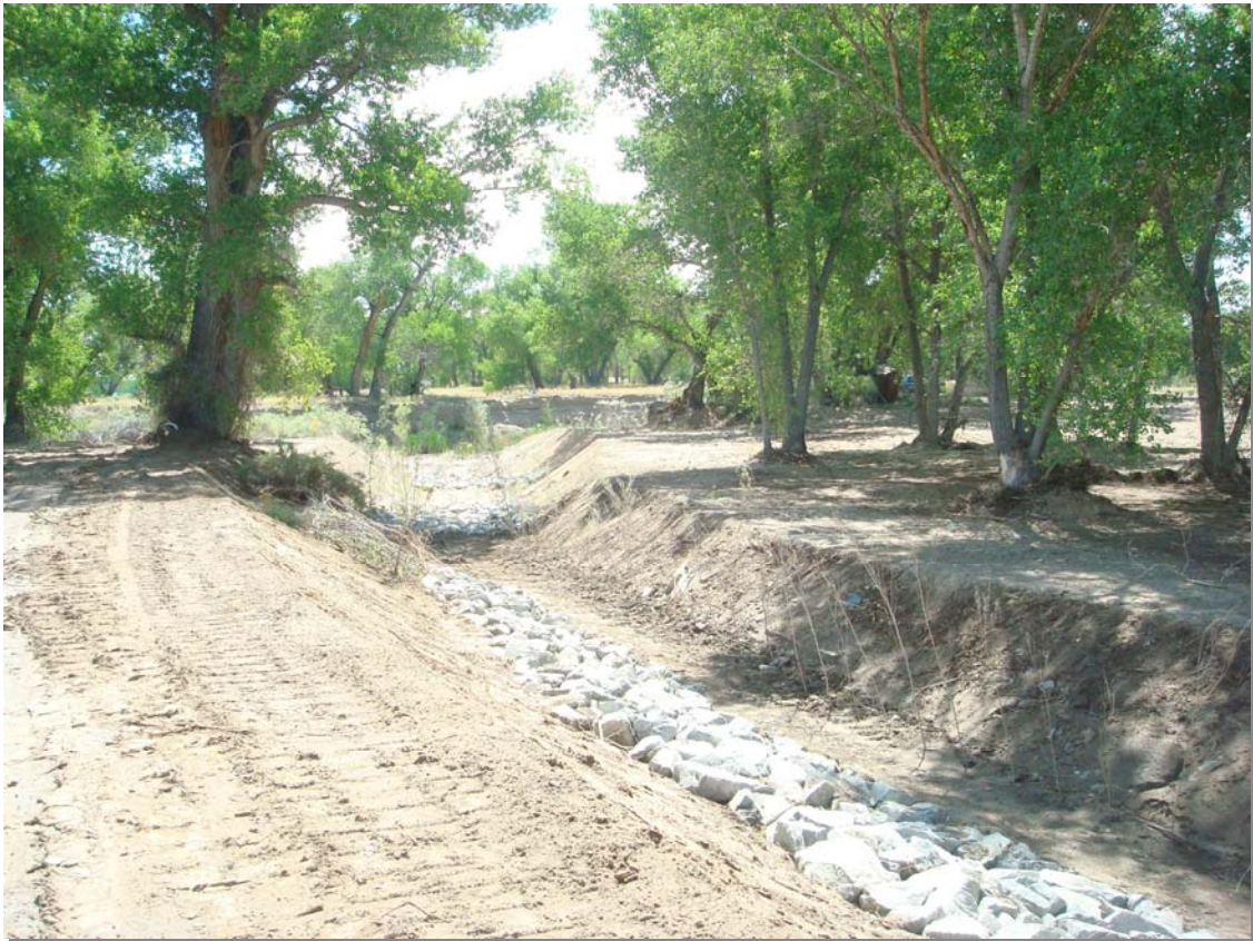
After Construction at Irrigation Return Flow Project
