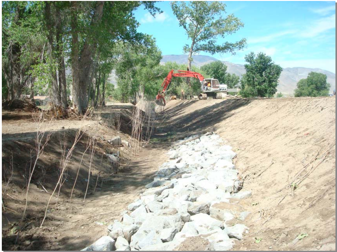
After Construction at Irrigation Return Flow Site
