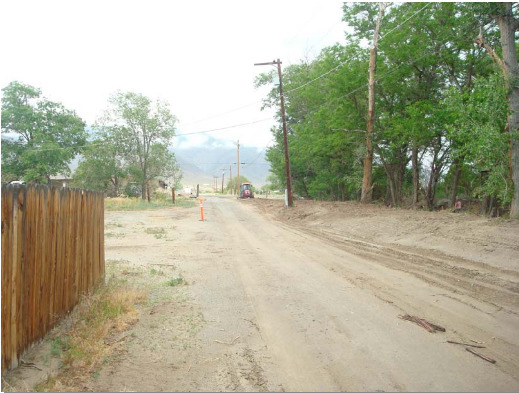
After Construction at Irrigation Return Flow Site
