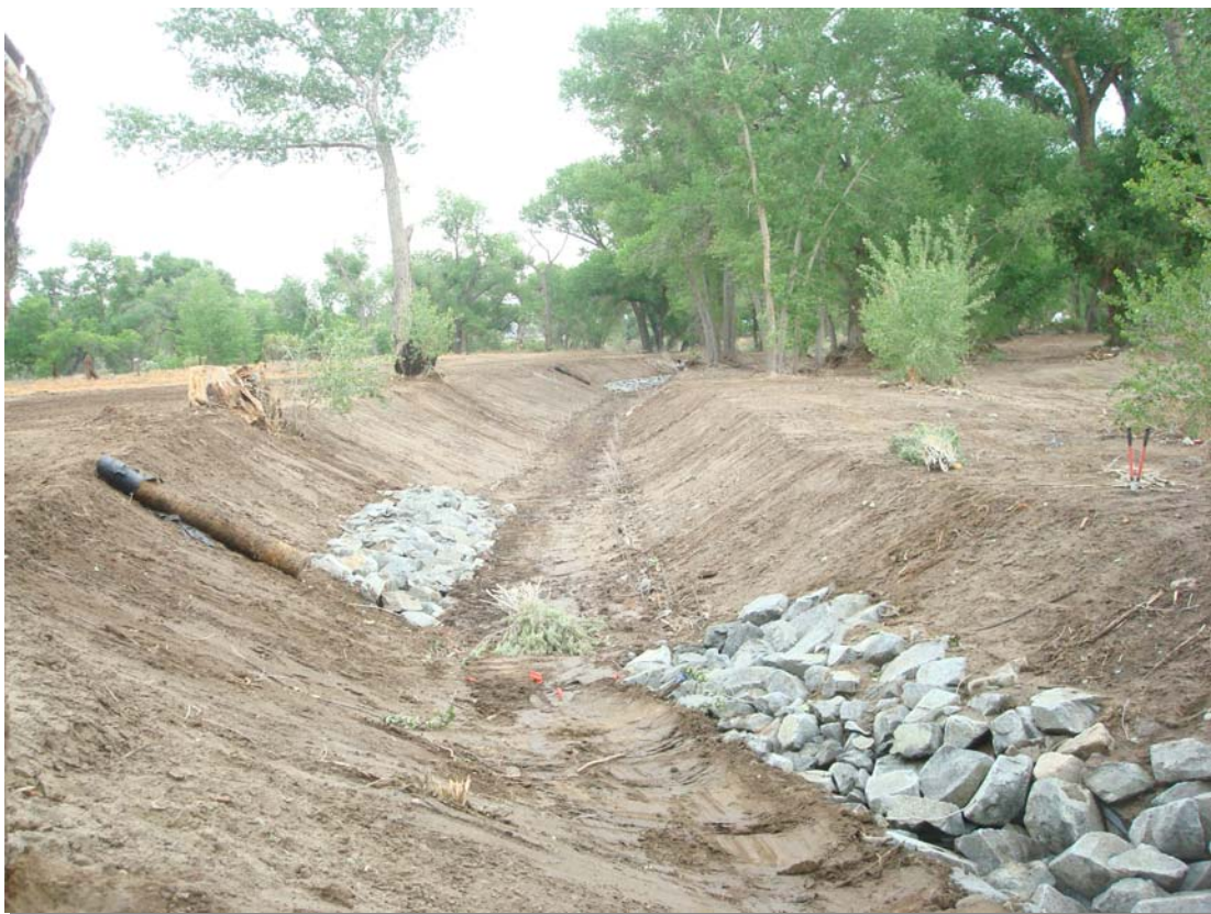
After Construction at Irrigation Return Flow Site
