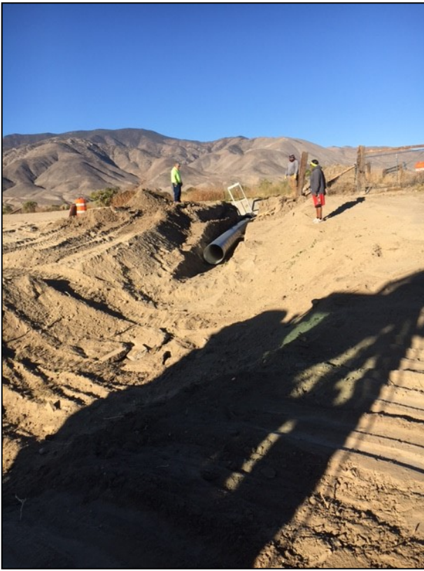
During Construction, Replacing Old Culvert with New Culvert
