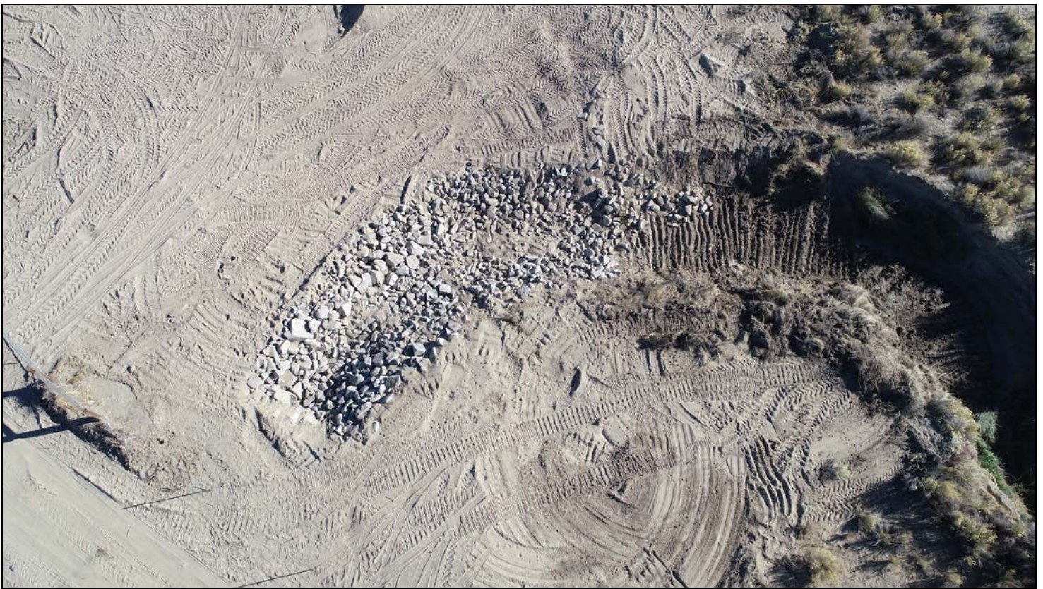
Finished Construction of Irrigation Return Flow Ditch, Top Aerial View
