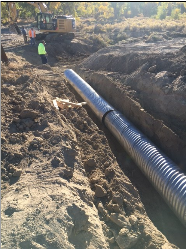
During Construction, Replacing Old Culvert with New Culvert
