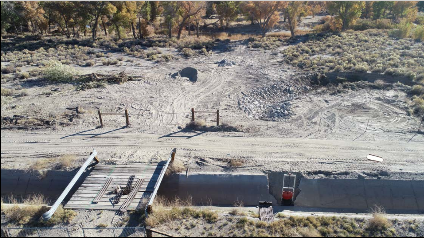
Finished Construction of Irrigation Return Flow Ditch, East Aerial View
