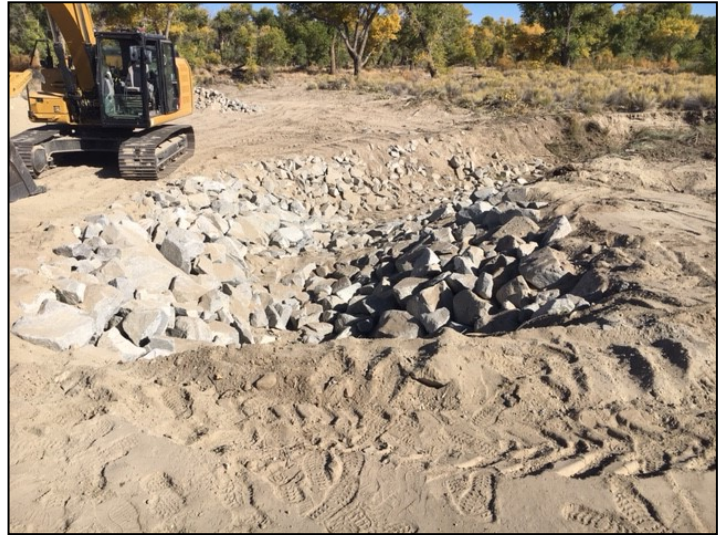
During Construction, Rip Rap Rock Delivery, Rip Rap Rock Placement in Repaired Ditch
