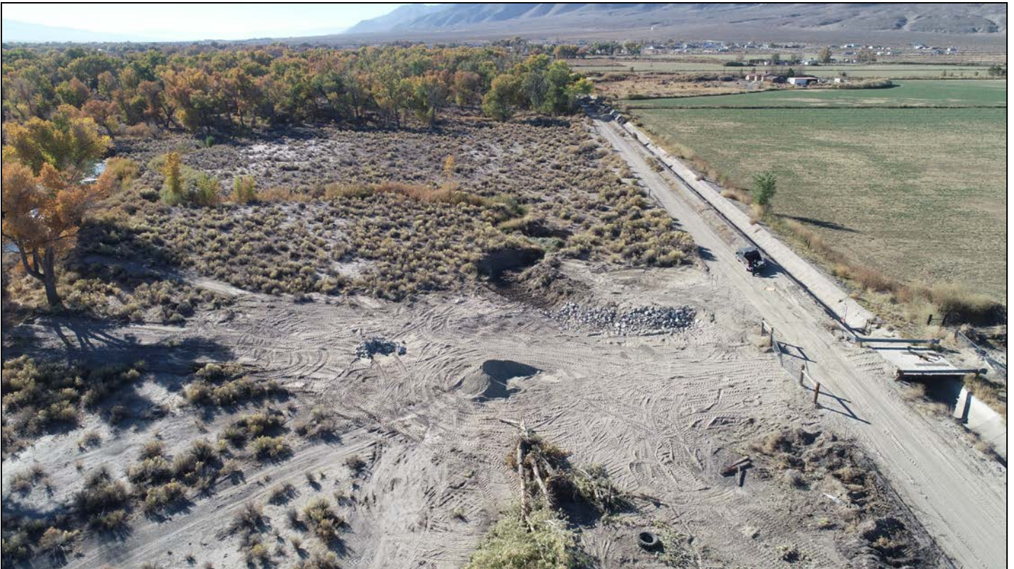
Finished Construction of Irrigation Return Flow Ditch, South Aerial View
