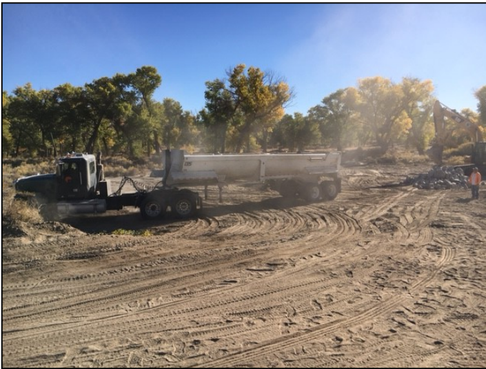
During Construction, Rip Rap Rock Delivery, Rip Rap Rock Placement in Repaired Ditch
